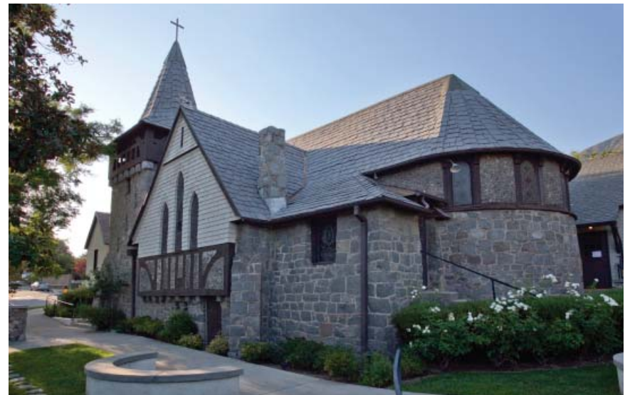
Episcopal Church of the Ascension Source: Seth Hanson
