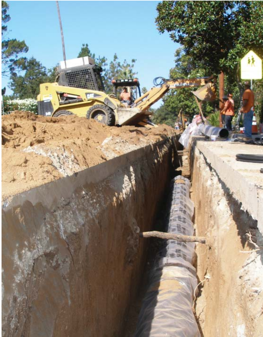
Sierra Madre Boulevard Water Main
