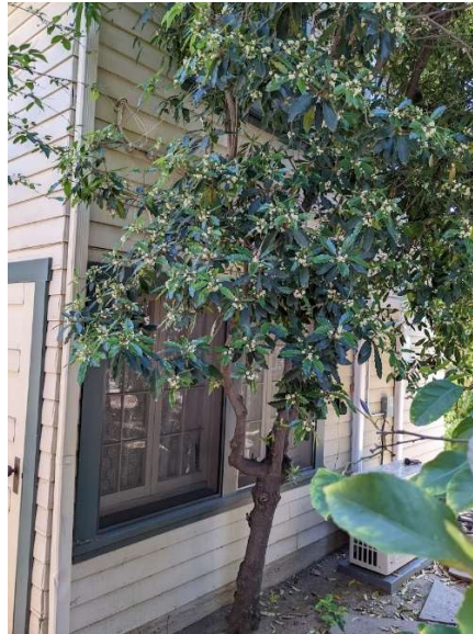
Side/Western Façade, 615 W. Montecito Avenue (view facing southeast)
