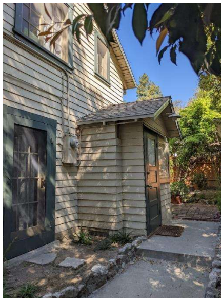
Side/Eastern Façade, 615 W. Montecito Avenue (view facing northwest)
