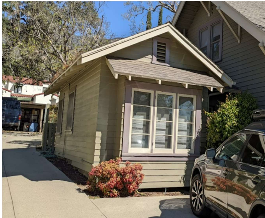
Southern Façade, 619 W. Montecito Avenue (abutting 615 W. Montecito Avenue)
