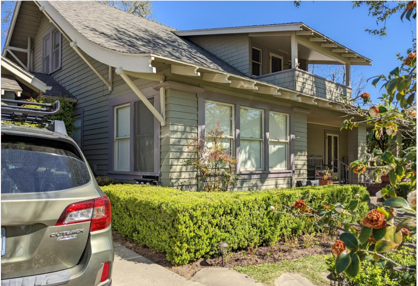
Primary/Southern Façade (view facing northeast)
