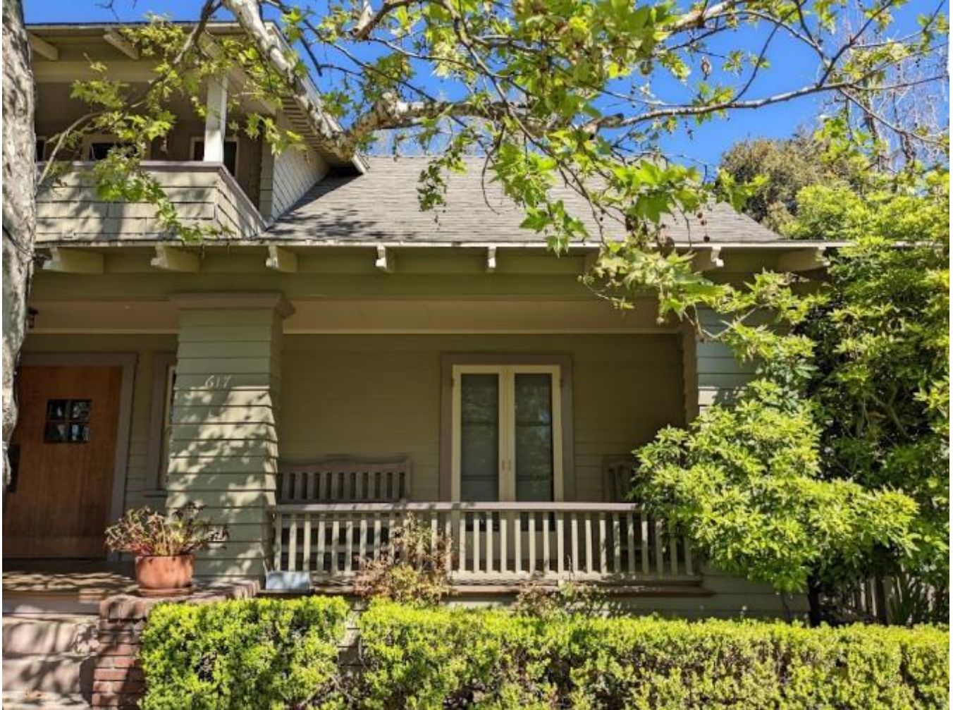
Primary/Southern Façade (central section)
