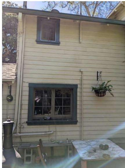
Side/Eastern Façade, 615 W. Montecito Avenue
