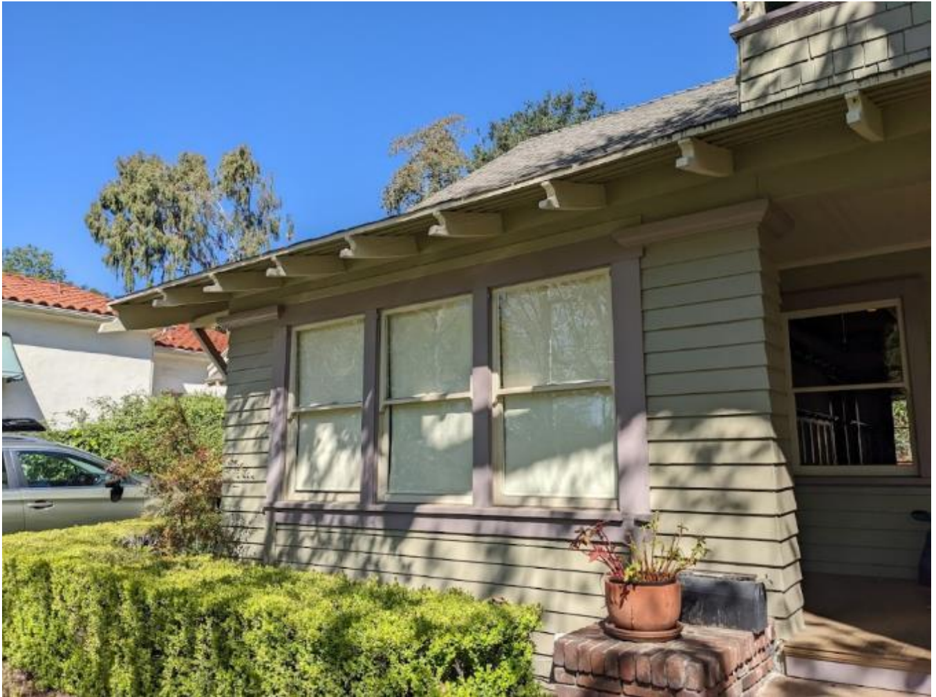
Primary/Southern Façade (left section)
