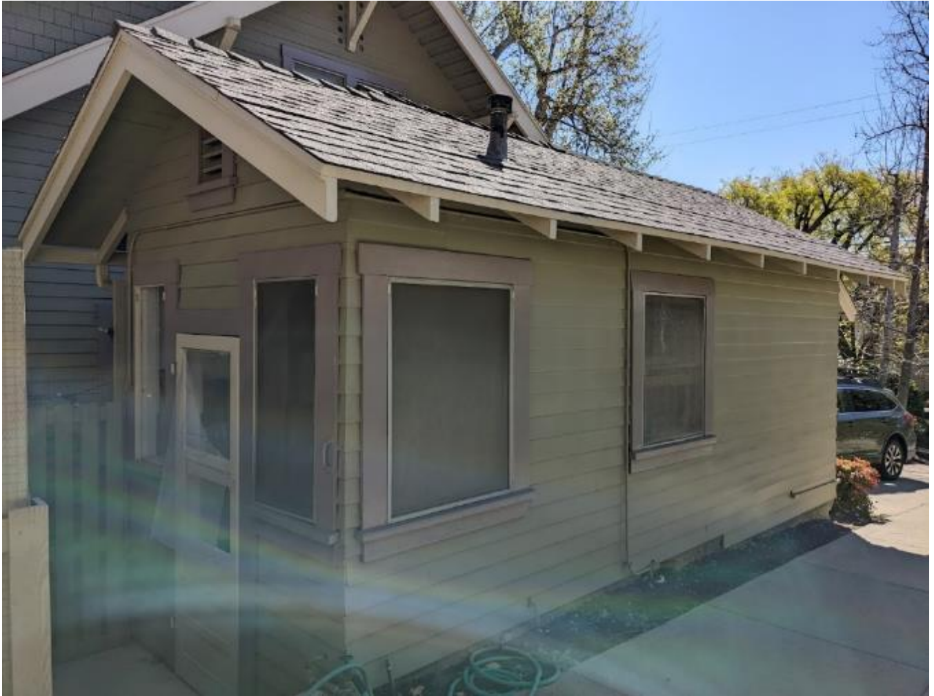
Northwest Corner (showing northern façade at left)
