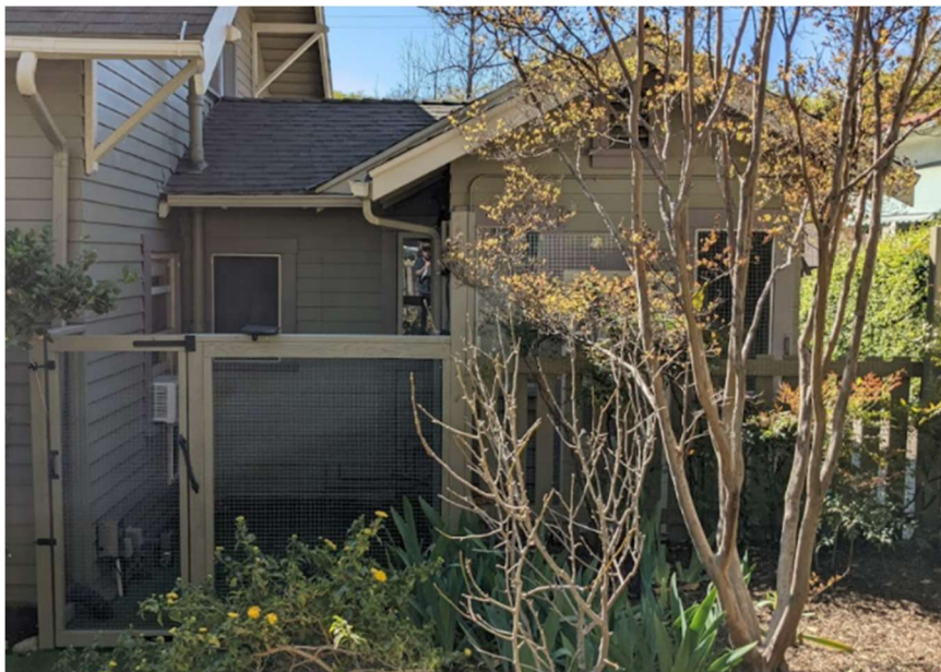
Rear/Northern Façade, 619 W. Montecito Avenue
