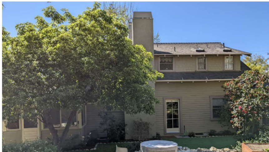
Rear/Northern Façade, 617 W. Montecito Avenue (main portion, excluding DPU)
