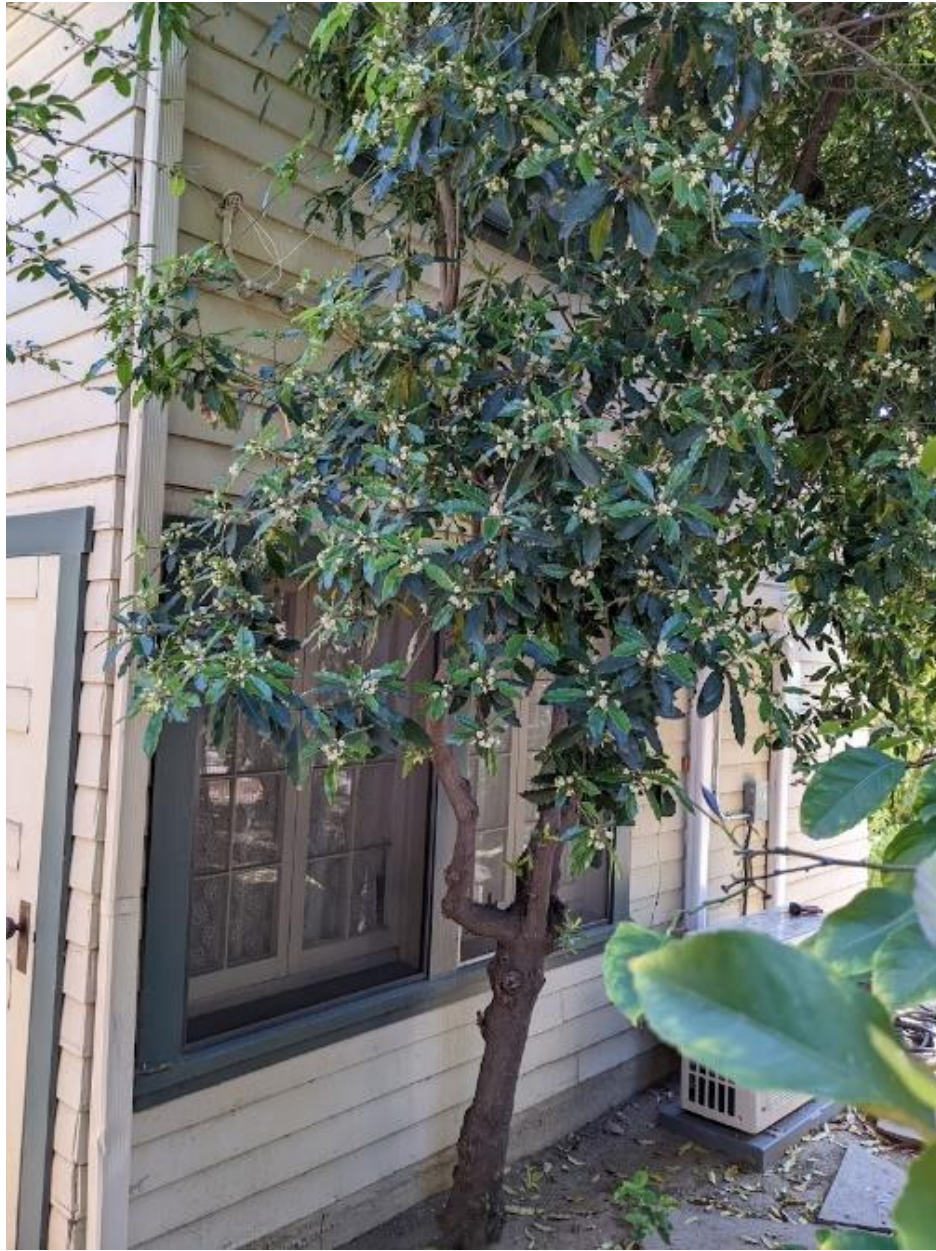
Side/Western Façade (view facing southeast)
