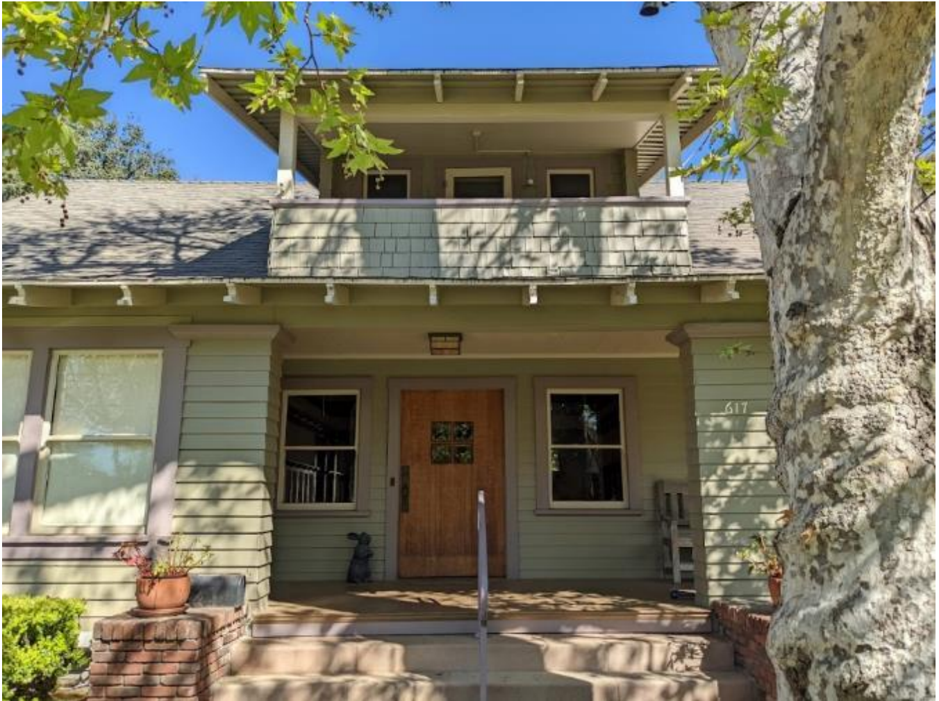
Primary/Southern Façade (central section)
