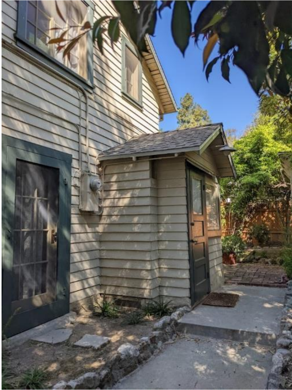
Side/Eastern Façade (view facing northwest)
