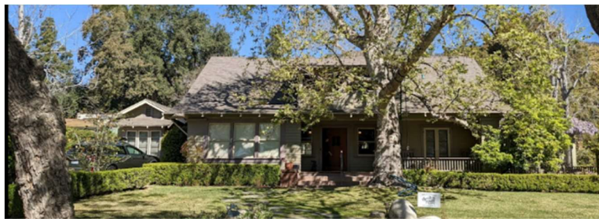
Primary/Southern Façade (617 W. Montecito Avenue at right; 619 W. Montecito Avenue at left)
