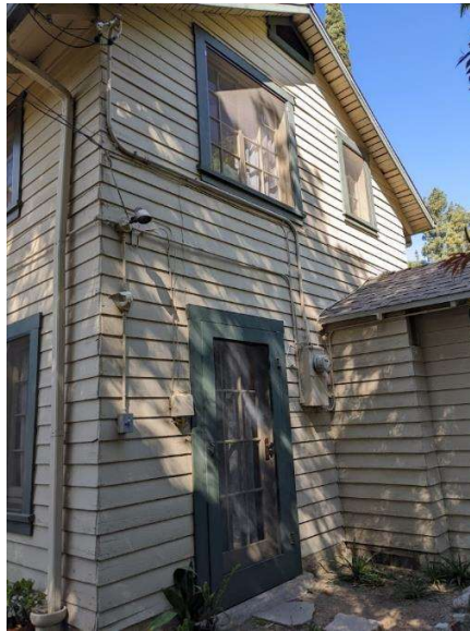
Side/Eastern Façade, 615 W. Montecito Avenue
