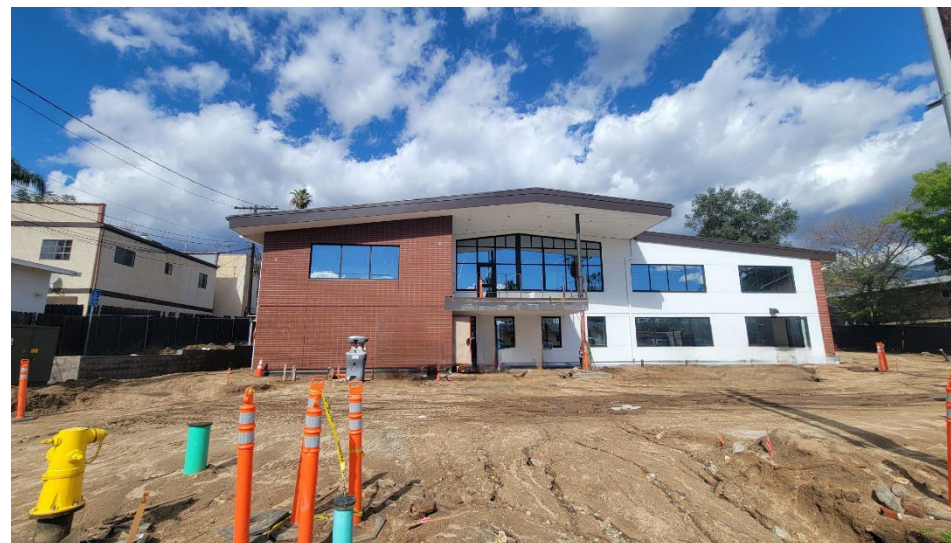
Sierra Madre Library Under Construction.
