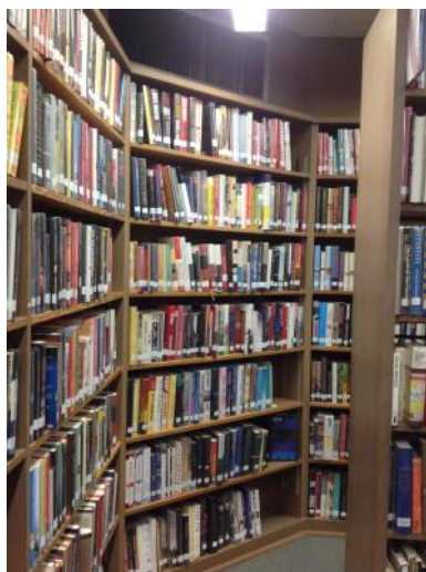
The current shelving placed at widths of 30” to 36” is too narrow to meet the 44” requirements in California code and ADA requirements. Shown below, the Library’s existing emergency exits are not acces-
